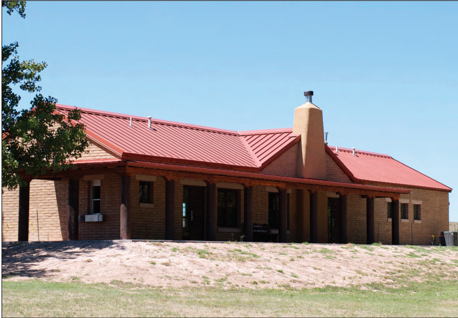
With the help of the Friends of Meade State Park, this visitor's center opened in 2007. The ADA-accessible facility is available for programs, meetings and family gatherings
