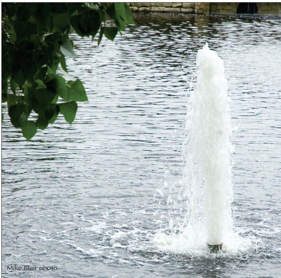
Aeration systems can be bubblers, pumps or fountains. Fountains are effective and can add an element of beauty to a pond, but they are the most expensive system to operate.
